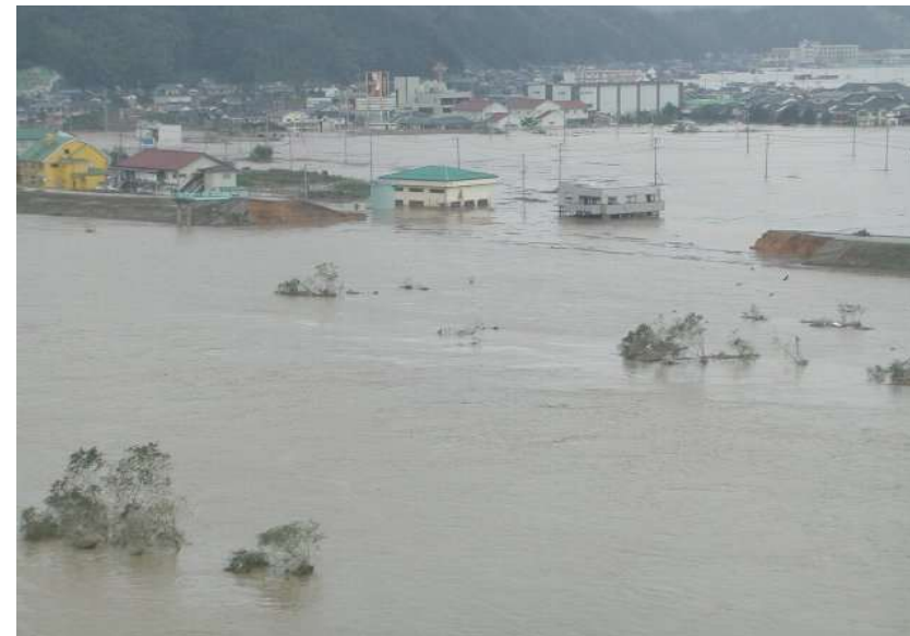
Broken embankment of the Maruyama River (Tateno, Toyooka City)
